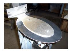
Back and inlet grille panels should only be fitted after all functional tests have been completed and verified (See Commissioning).
